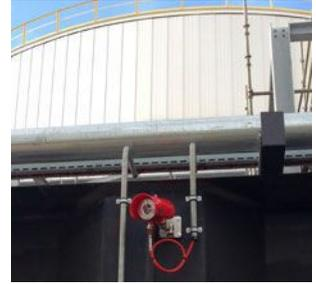
The Spectrex SharpEye Optical Flame Detectors used are Triple IR Optical Flame Detectors, providing accurate fire protection with high false alarm immunity. The SharpEye 20/20SI Triple IR Flame Detectors were installed in the first phases and SharpEye 40/40I Triple IR Flame Detectors in the next phases. In total, over 60 of these Triple IR Optical Flame Detectors have been installed at the terminal.
